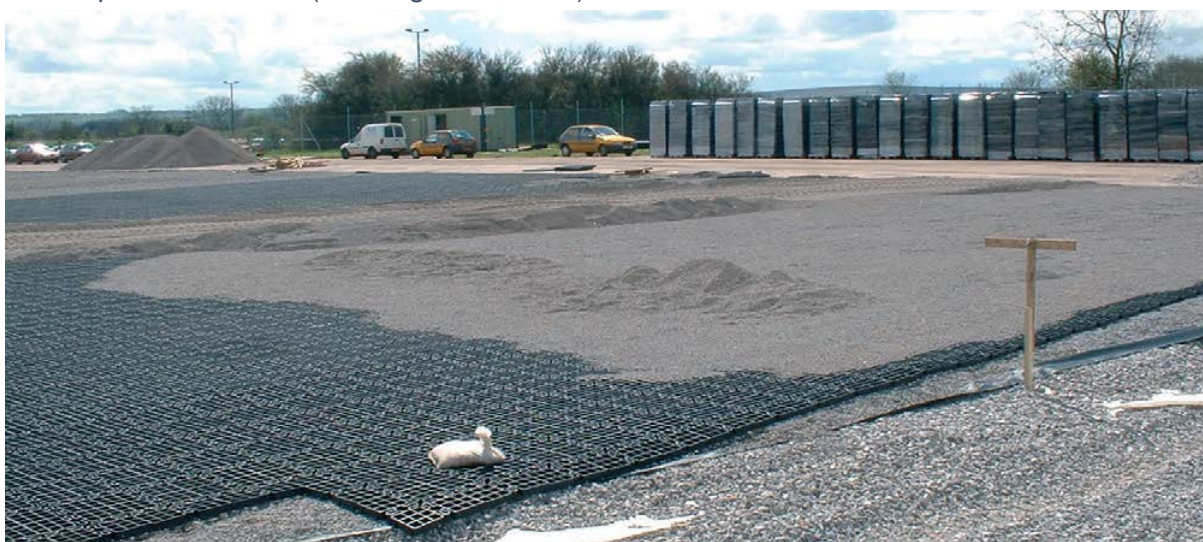
Figure 4.9: Bristol International Airport car park covered in permeable paving using the Netpave 50 system discharging into swales (Bristol.gov.uk, 2016)
