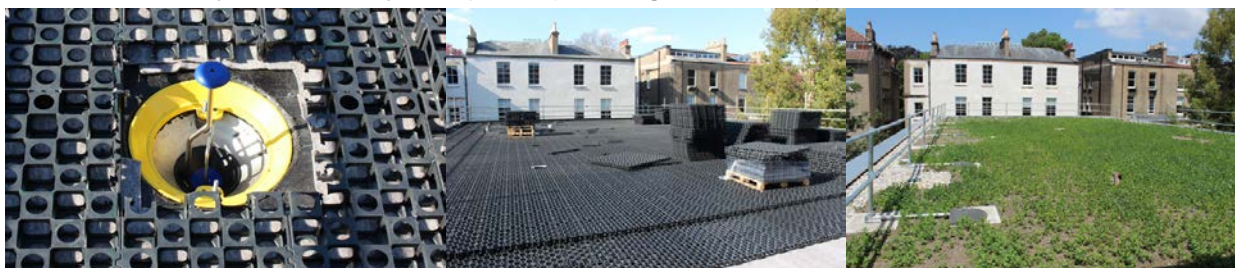
Figure 4.10: Blue and green roof at Bristol University Auditorium (Bristol.gov.uk, 2016)
